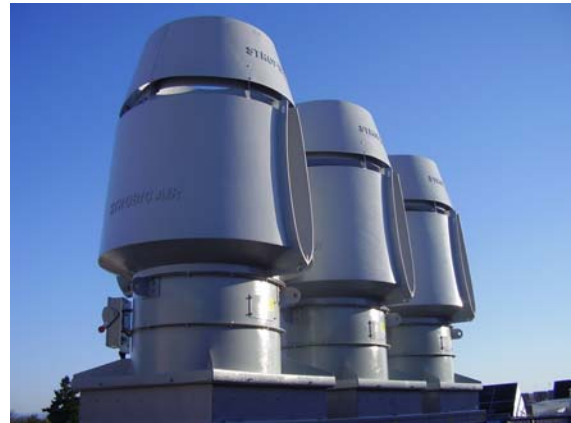
Installing the variable speed fans to replace single speed fans for the building. 12,000 pounds worth of metal!
