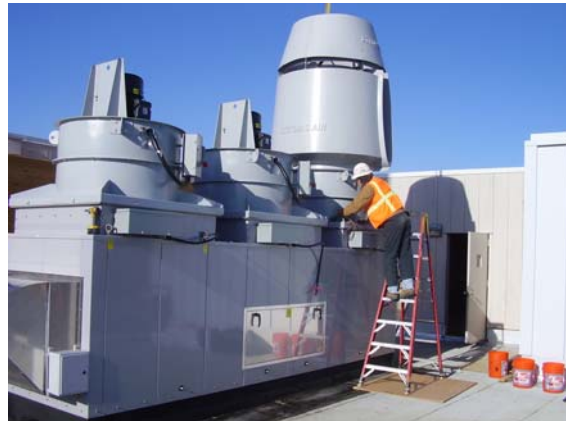
Installing the variable speed fans to replace single speed fans for the building. 12,000 pounds worth of metal!
