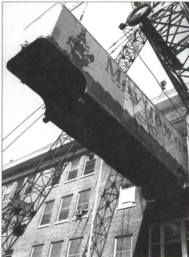
Moving day, June 8, 1970, with the moving van trailer raised to the fourth floor of Agriculture Hall.
